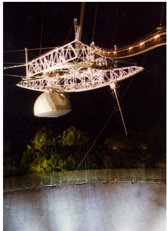
Arecibo Observatory at Night courtesy of the NAIC - Arecibo Observatory, a facility of the NSF
